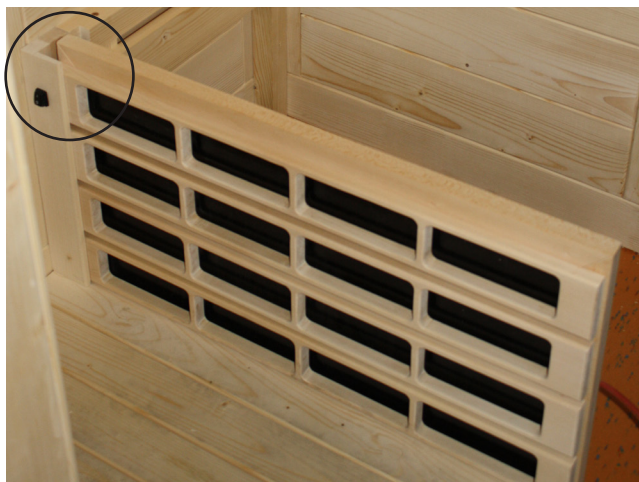
Fig. 34: Installation of the IR thermal plate VitaMy 164
