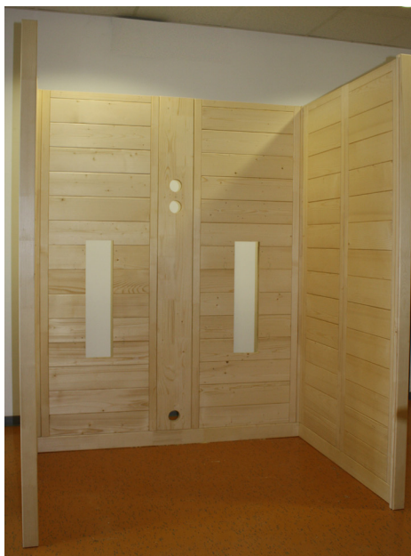
Fig. 10: Installed wall elements
