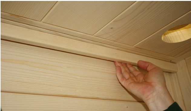
Fig. 38: Glueing the LED strips in place
