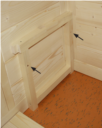
Fig. 32: Installation of the bench cushion
