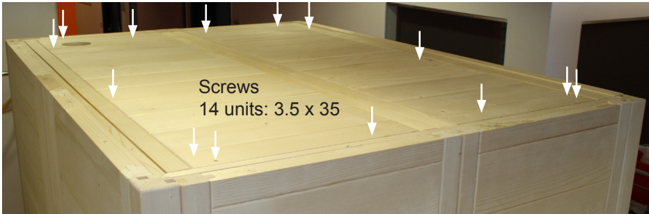
Fig. 19: Attaching the roof element
