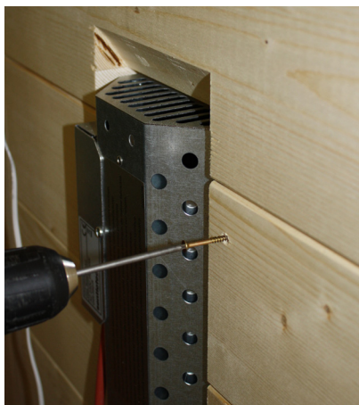
Fig. 42: Installing the rear radiator blind
