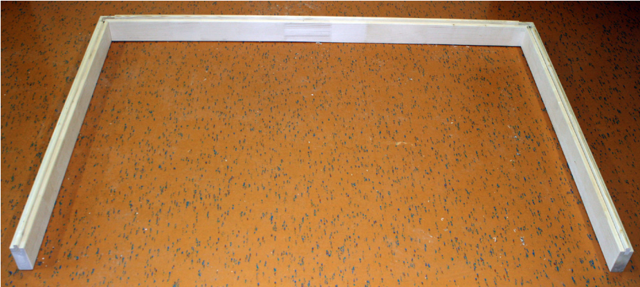
Fig. 1: Placing the three floor frame elements
