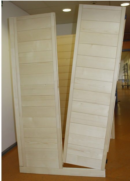
Fig. 9: Installation of the two front corner posts with a groove for glass
