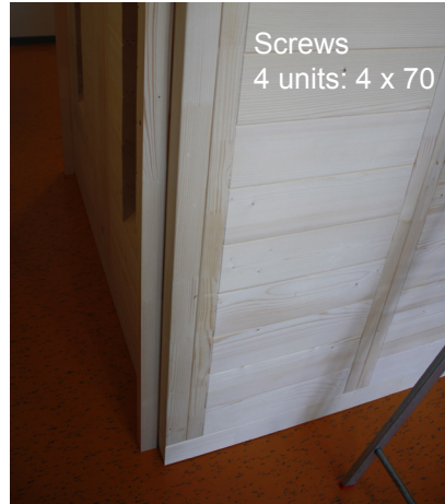
Fig. 52: Installation of the spacer strips of the rear wall
