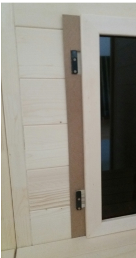
Fig. 53: Installing the backrests of the bench
