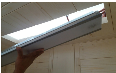
Fig. 50: Installing the colour light
