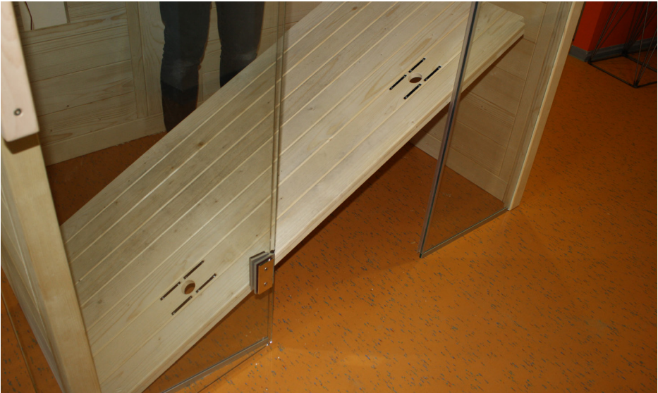
Fig. 28: Put the cabin floor in place
